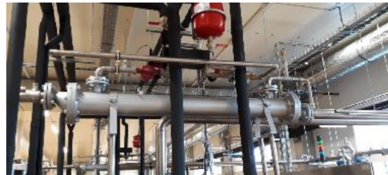
Decrystallization units DH 250, placed above tempering machines
